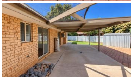
Unit 2, 3 Hume Street, Cobram
