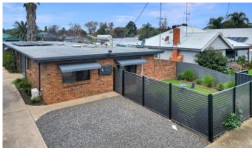
Unit 1, 6 Thompson Avenue, Cobram
